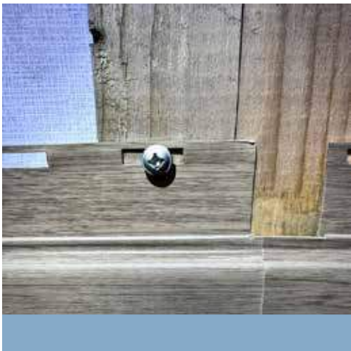
Figure 2 Properly gapped screw set evenly, level and square to the panel - see "Additional Considerations" section for more detail on fastening
