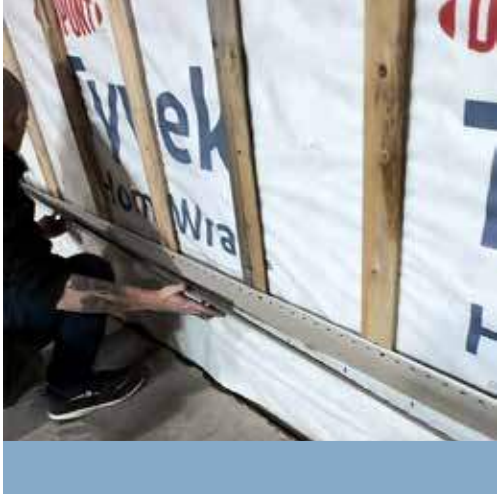
Figure 1 Hooking ALUZION Base Profile into Vented Starter Strip
