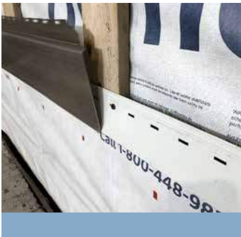
Figure 3 Hooking ALUZION Base Profile and applying even vertical pressure to set panel evenly into the starter strip.
